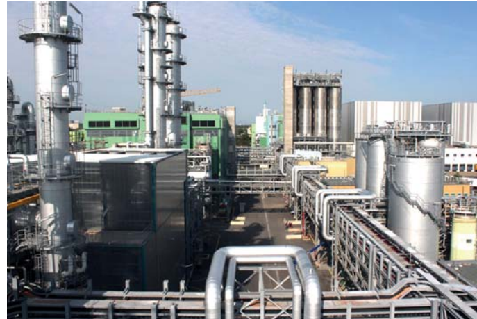
Production plant for high-performance plastics, Celanese
