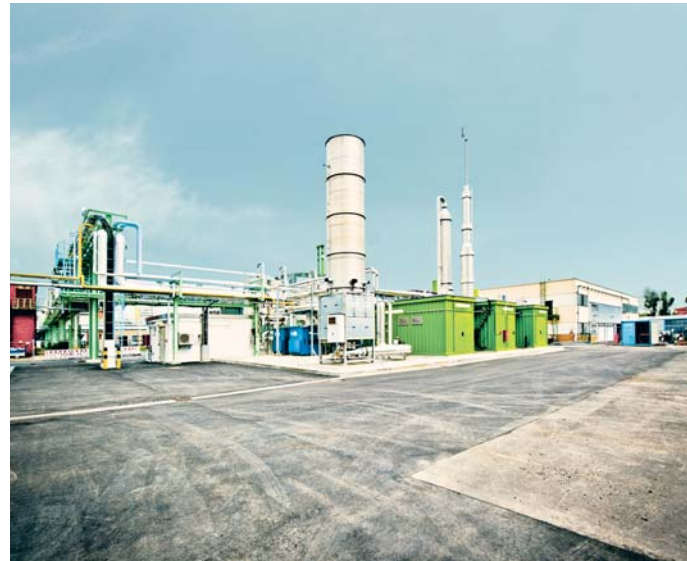
Biomethane upgrading plant, Infranova
