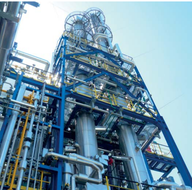
Dimethyl ether production facility, Grillo
