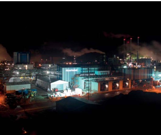
Expansion of chlor-alkali production plant, AkzoNobel
