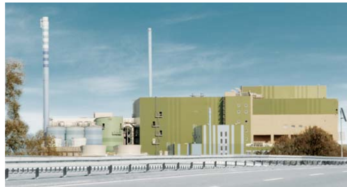
Waste-to-energy plant, Infraserp Höchst
