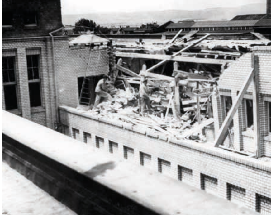
The auditorium was destroyed on June 29, 1940 by high-explosive bombs.
