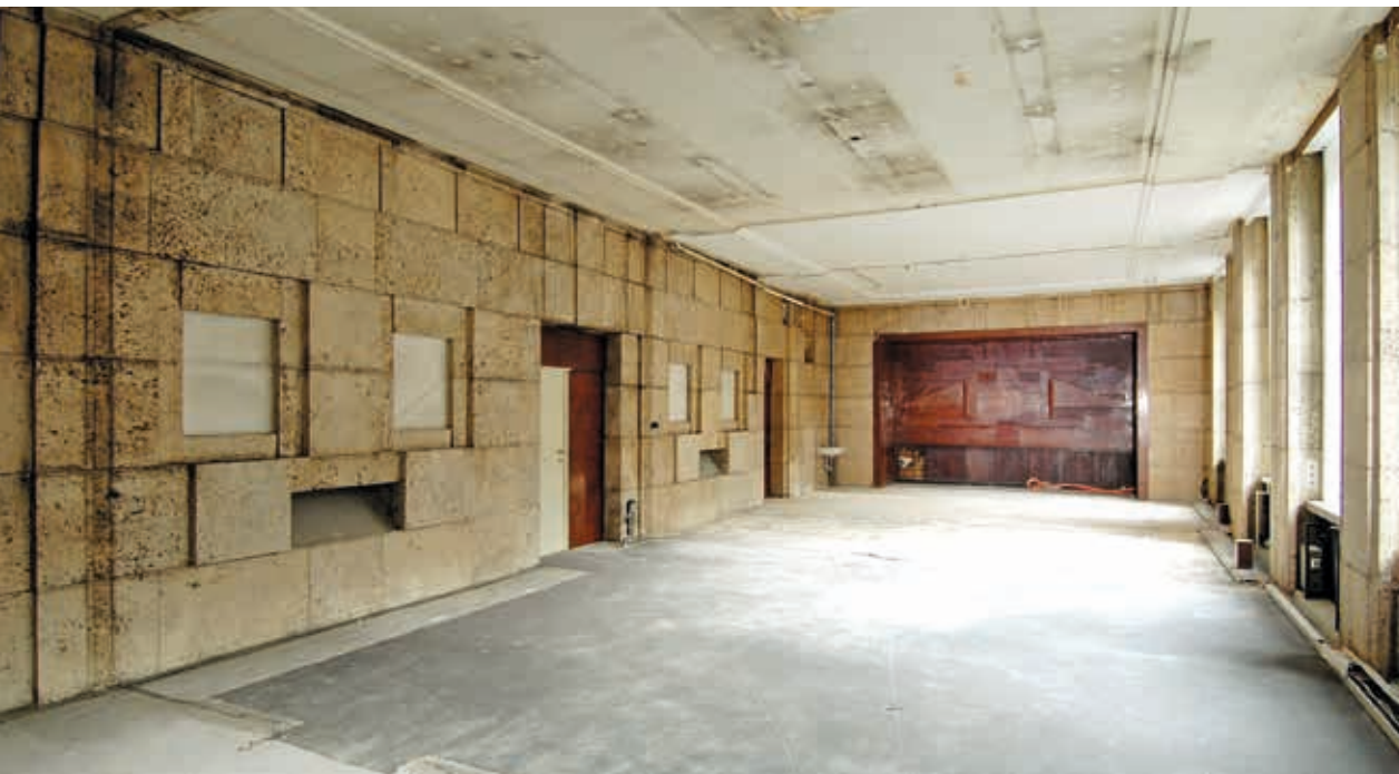
Removing the false walls in the Marble Room revealed the intact travertine cladding hidden underneath.
